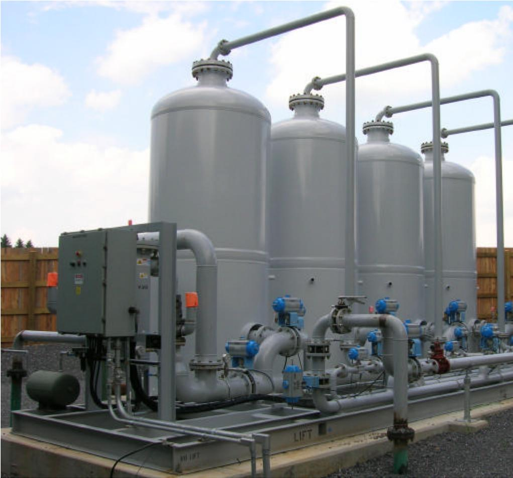
*Figure 2: Typical installation for a 2~ 4 MM SCFD Molecular Gate nitrogen rejection unit*
