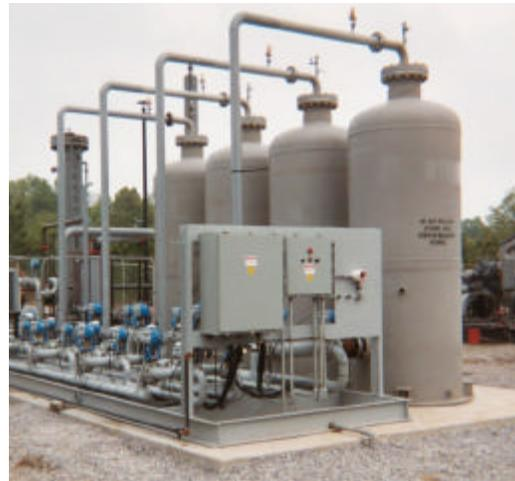
**Figure 6.** A 2.5 MM SCFD unit designed to upgrade CMM (plus contaminated natural gas)
